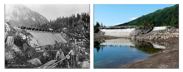
A 15-foot tall wooden dam was installed at the natural outfall of Upper Annex Lake during construction of the hydro project to allow more water to be stored. The dam failed in 1935 and was replaced the next year with a 20-foot tall dam. The dam was replaced again in 1967, and that dam stands today.
